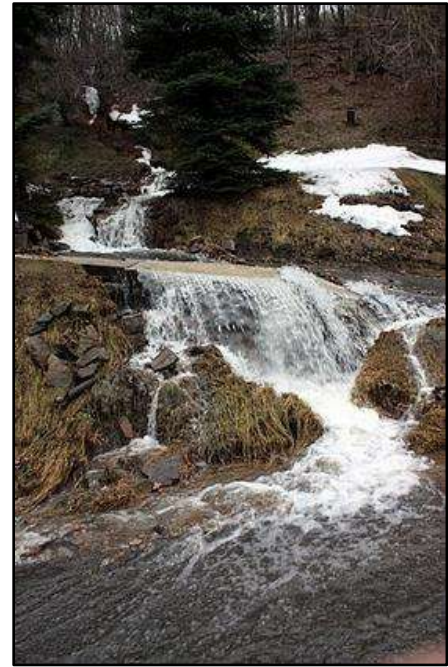
Figure 12-2. Flooding on Douglas Avenue. Source: Allegany County Department of Emergency Services.
